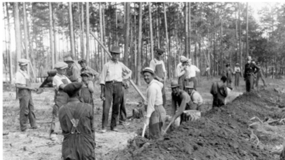
SGT. YORK, CENTER, DIGS FOUNDATION FOR YORK INSTITUTE
