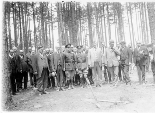
GROUNDBREAKING FOR YORK INSTITUTE
