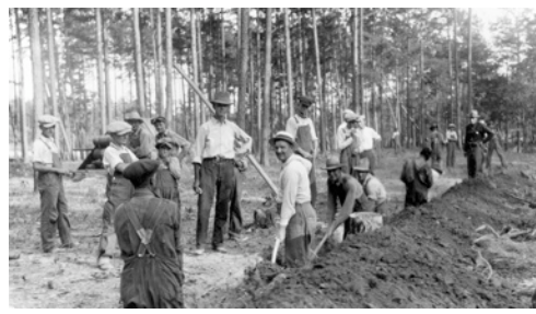
SGT. YORK DIGGING FOOTER FOR YAI IN WHITE SHIRT, CENTER
